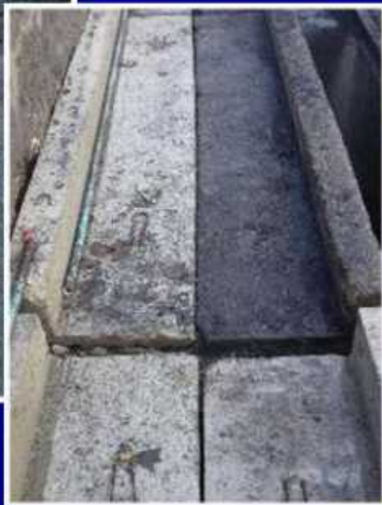
■ Repaired working ways: elements replaced.
